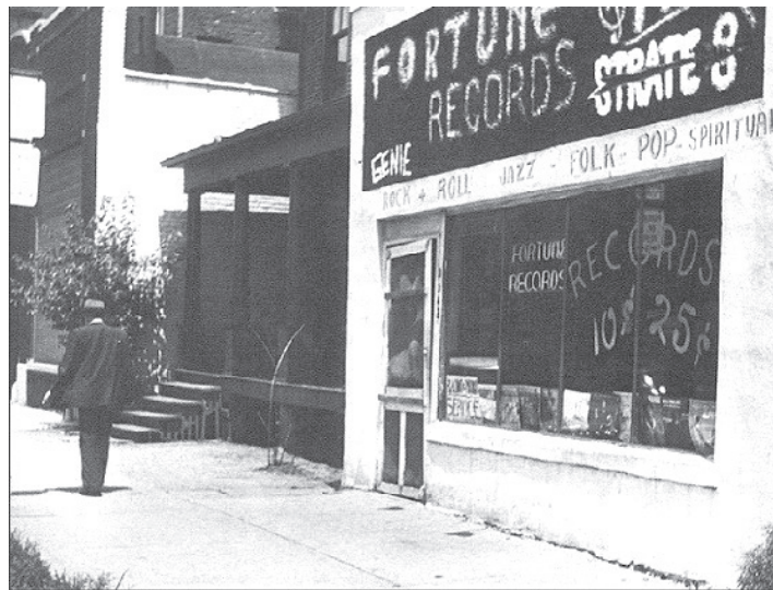
Fortune Records building at 3942 Third Ave., Detroit Michigan. It was demolished in 2001 after years of vacancy.
